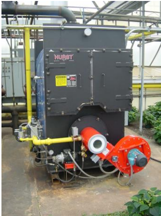
• Dual fuel boiler (natural gas & fuel oil)
